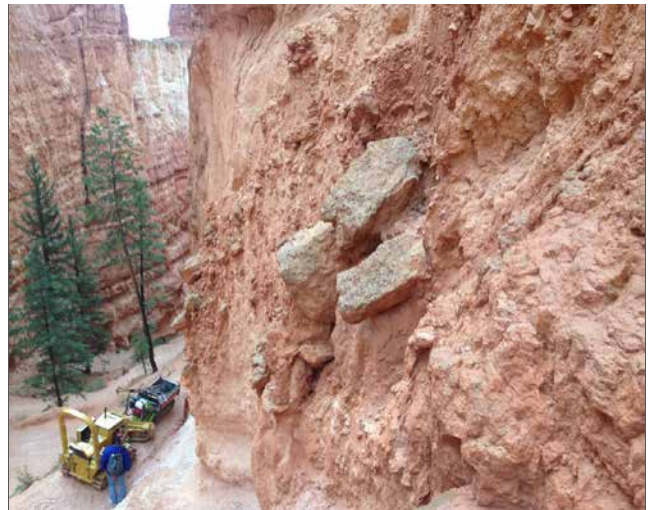
Figure 4.5.4-1. Rockfall hazard along the Navajo Loop Trail. Photo Credit: NPS.
