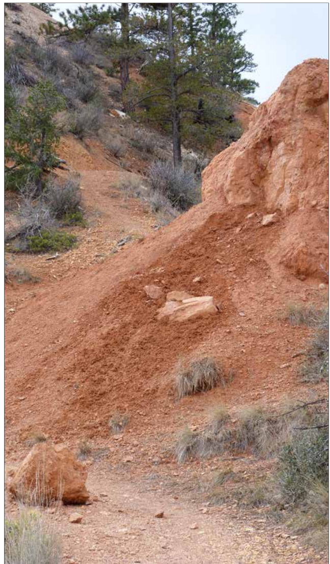
Figure 4.5.4-2. Rockfall along the Fairlyland Trail. Photo Credit: NPS.
