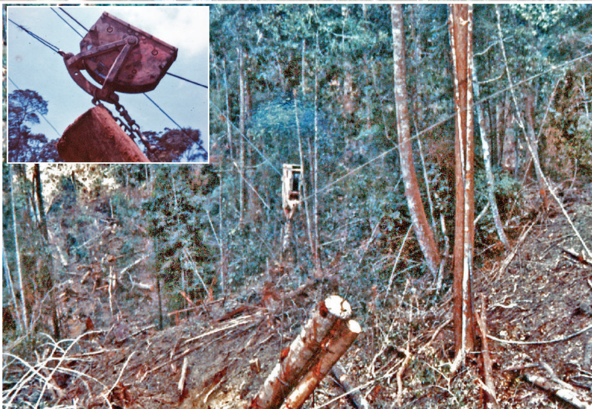
Fig.13. Scooter turn approaching landing, North Borneo Timbers c.1978. (Photo Ross Ibbotson) The perspective shown in this view is deceptive; the remote landing was at least 2000 ft from, and 600 ft below, the roadside. (Inset) Fig. 12: Close up of NBT Scooter Carriage (Photo Ross Ibbotson).
