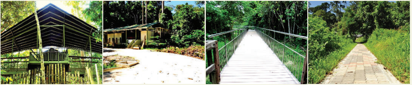
(L-R) Front view of the observation platform; concrete road to the new bear house; access boardwalk connecting the main Sepilok car park with BSBCC; and ground path leading towards the future BSBCC visitor centre.
