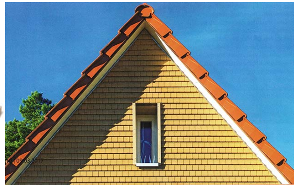
Figure 4. Facade, wooden shingles [source: 8]
