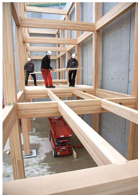
Figure 5. Support structure construction from beech [source: 10]
